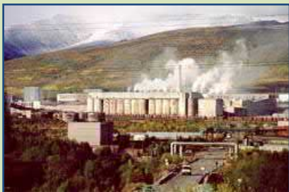
1. The Kovdor Dressing Plant
