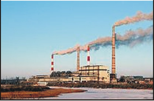
Dust from two heat power plants
