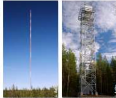
Instruments on mast (130m) and towers to measure at different heights
